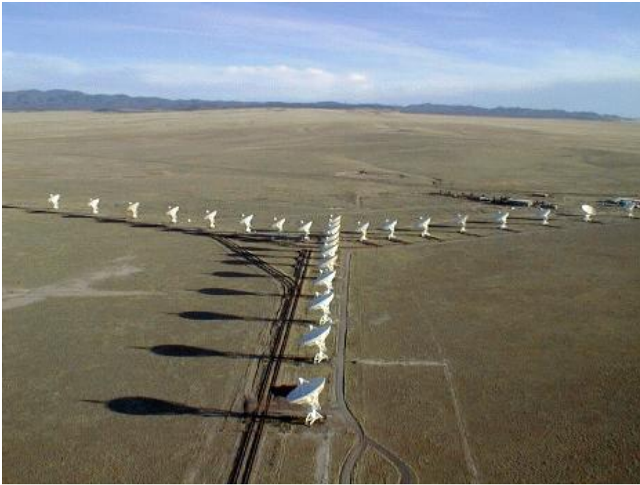
Figure 1. The Very Large Array in its Most Compact Configuration
